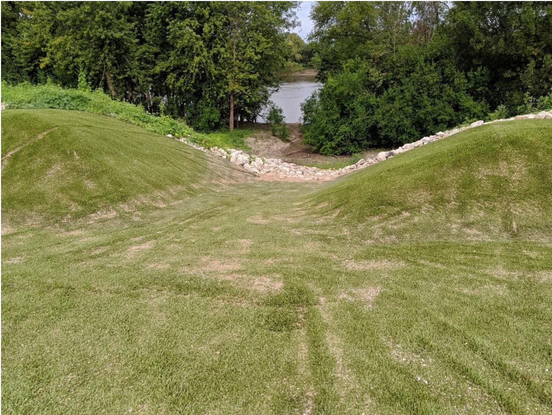
Photograph 3 ▲ - View of sand present in typical downlet structure, looking northwest.
