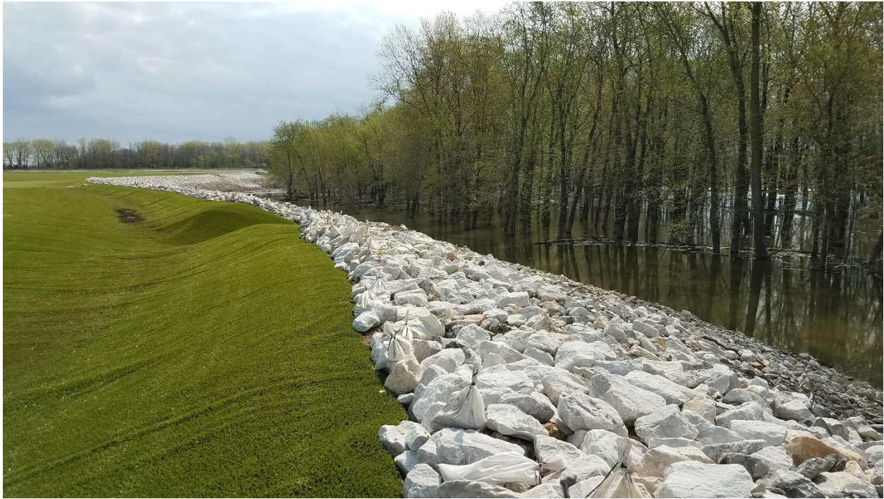
Photograph 1 ▲ - View of flooding near the Fly Ash Pond area, looking east.
