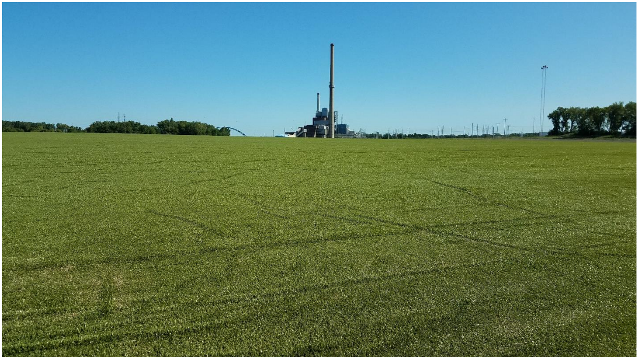
Photograph 6 ▲ - Typical view of final ClosureTurf cover, looking northeast.
