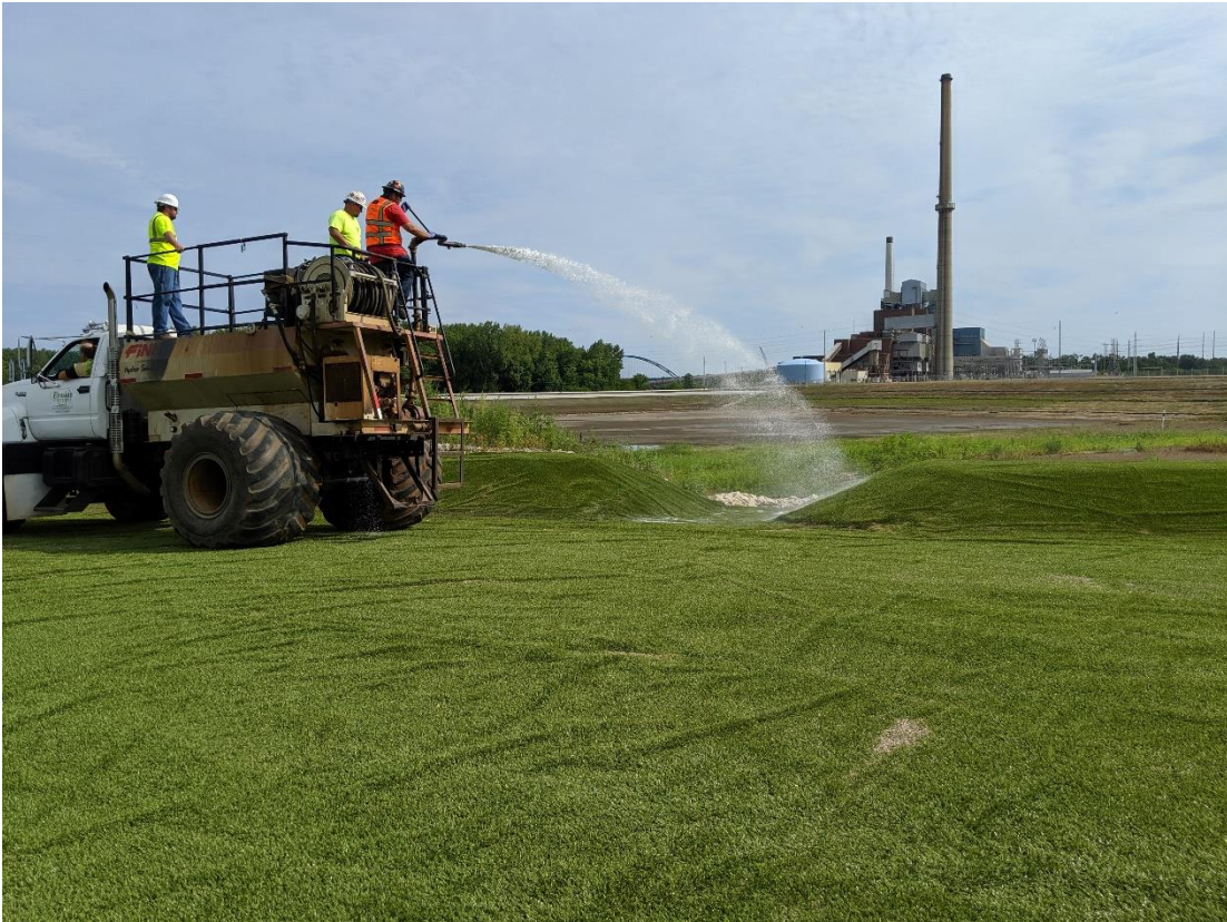
Photograph 4 ▲ - View of Armorfill placement activities, looking northeast.
